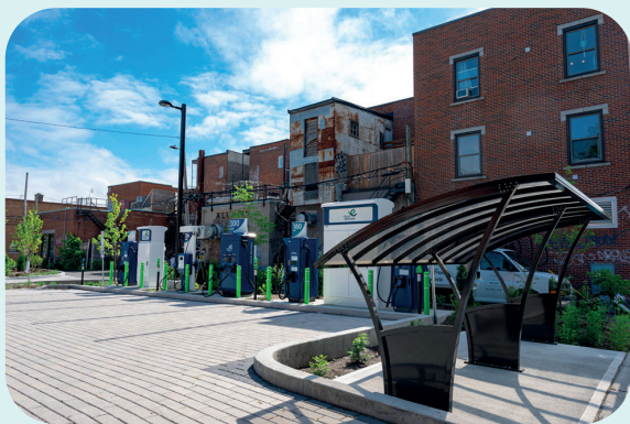
→ EV Fast Charging Stations and Covered Bike Parking
